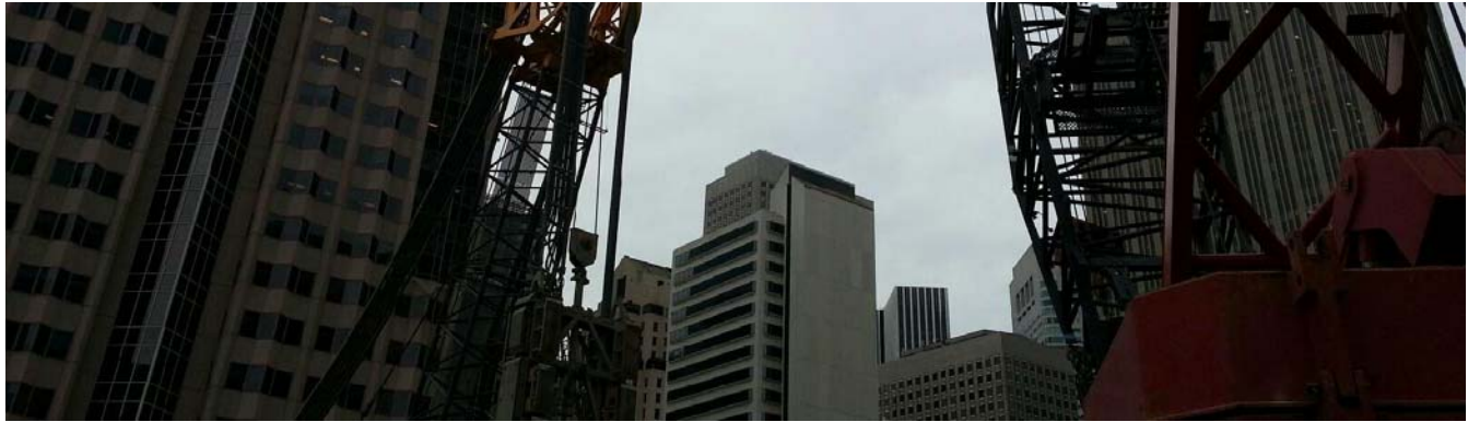
View of the San Francisco Skyline from the Transbay Tower Job Site
