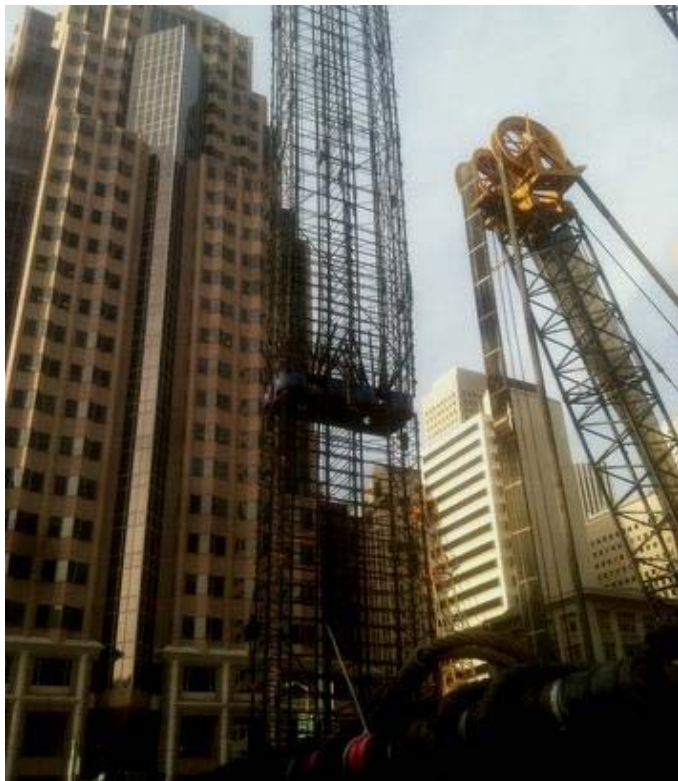
Lower Rebar Cage with O-cells Lowered into Excavation
